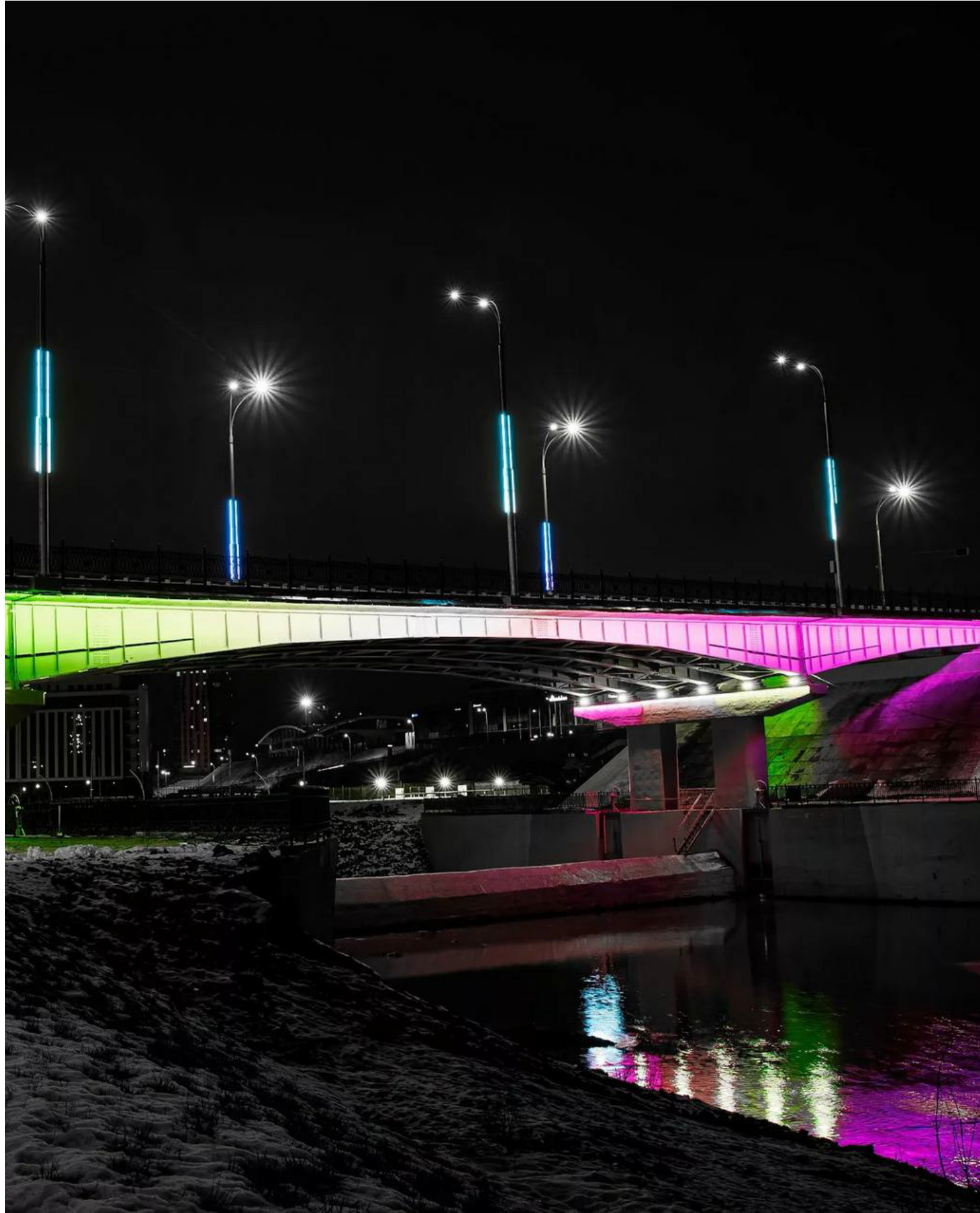
UNIVERSITY BRIDGE KEMEROVO
